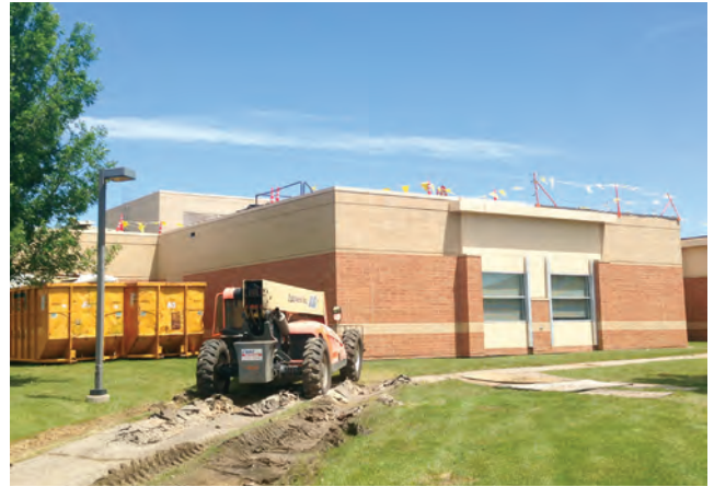
Figure 2. Roof replacement in progress
