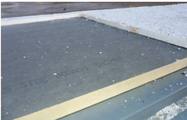
Figure 3. Existing roof being removed
