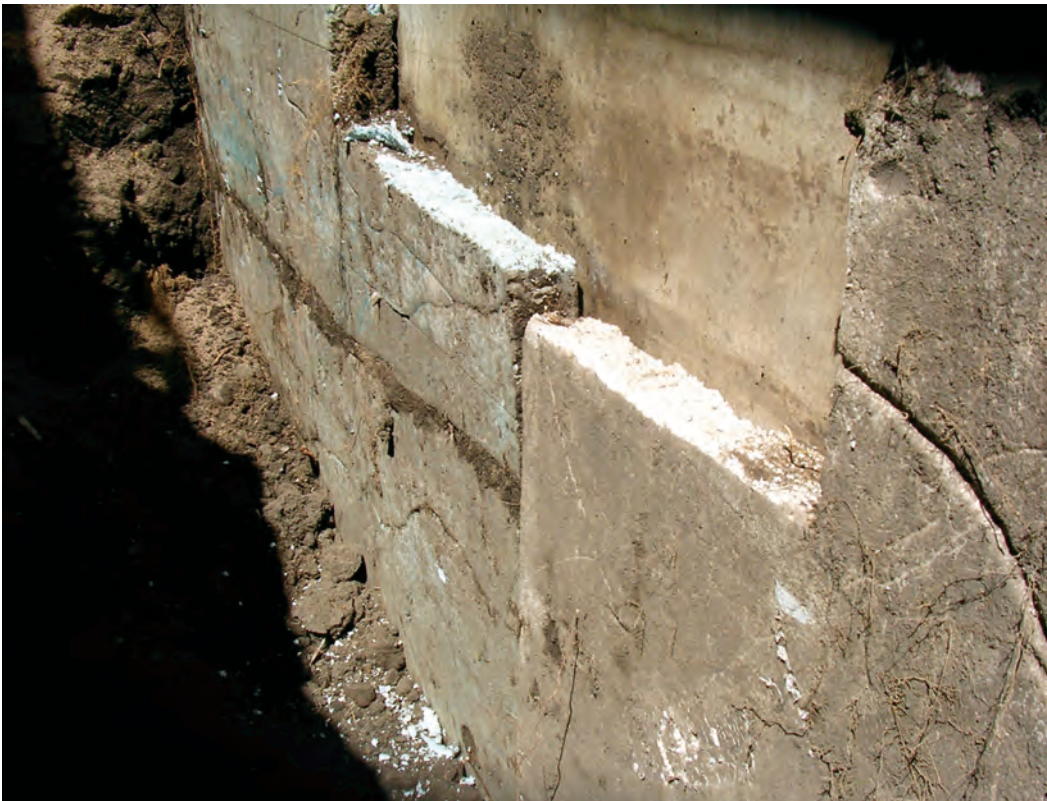
Figure 2. XPS and expanded polystyrene below grade insulation
