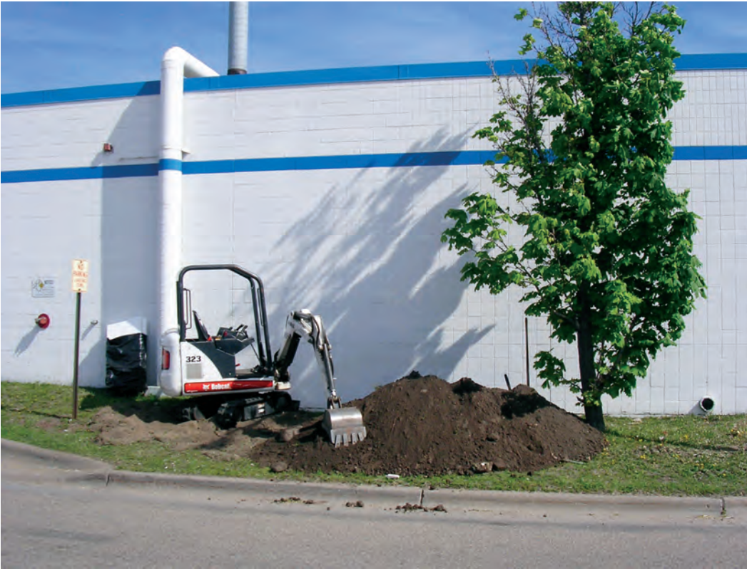
Figure 1. Excavation of insulation samples after 15 years
