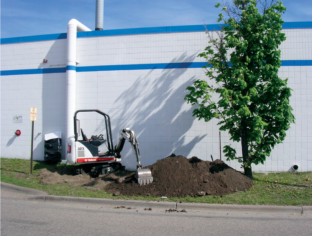
Figure 1. Excavation of insulation samples after 15 years
