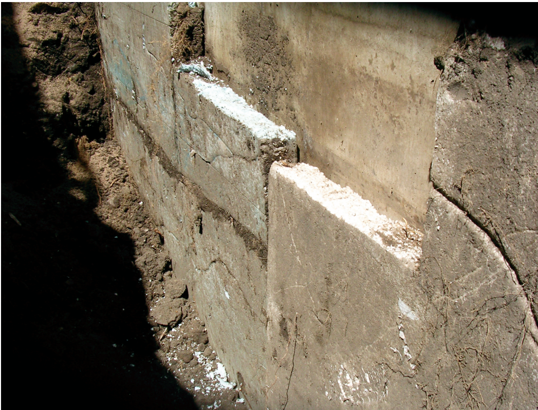
Figure 2. XPS and expanded polystyrene below grade insulation
